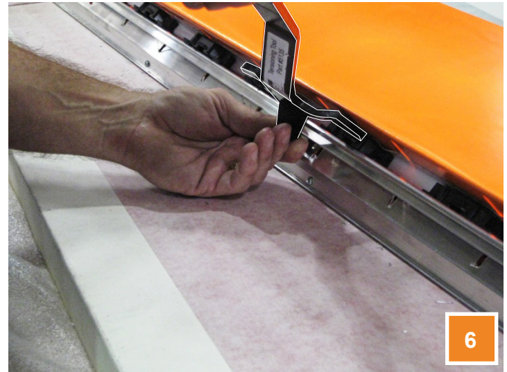
Use the tension tool to finish tightening the face. Be sure to alternate between top and bottom sides to keep the face even and installed properly.
